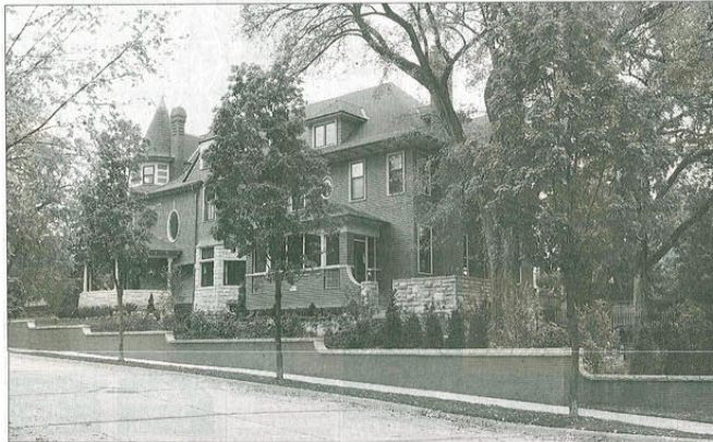
The contractor first removed about 16 feet from the back of the house before building a seamless four-story addition that begins at the side screened porch. It includes a family room and kitchen, a master suite and children's playroom.
