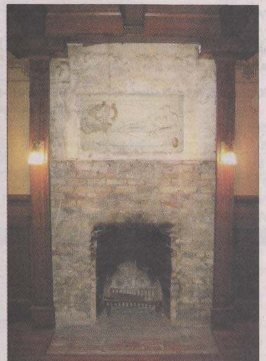
BEFORE: Demolition of the existing fireplace's drywall and marble slab, left, revealed the original brick facade and plaster bas relief panel, right.
