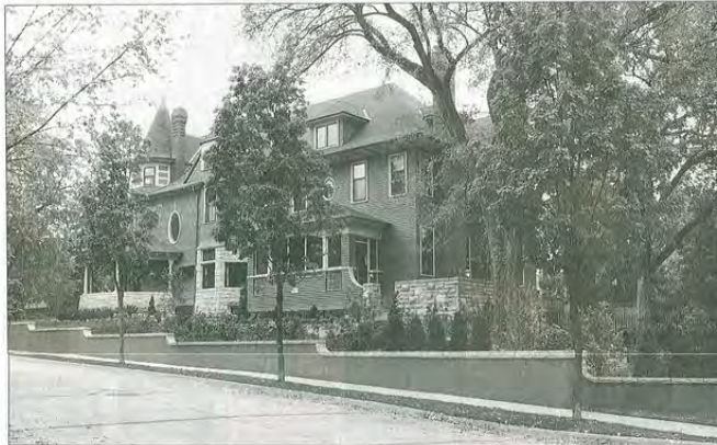
The contractor first removed about 16 feet from the back of the house before building a seamless four-story addition that begins at the side screened porch. It includes a family room and kitchen, a master suite and children's playroom.
