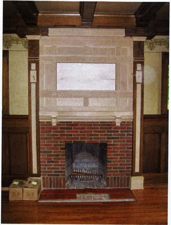
CLOCKWISE, FROM TOP LEFT: Behind the drywall, the owners found a classical bas-relief panel. The cabinetmaker created a new overmantel treatment and reconfigured the pilasters to accommodate vintage sconces, which now illuminate the sculpted frieze. Conserved and repaired, the panel is framed by the woodwork.
