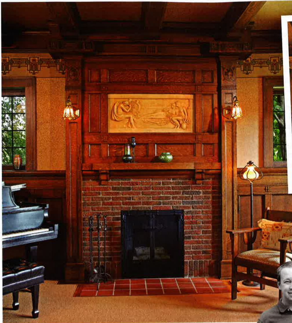
Restored to glory—with original bricks in the surround. A new overmantel took the place of damaged bricks under later drywall. The bas-relief panel was found under the drywall.
